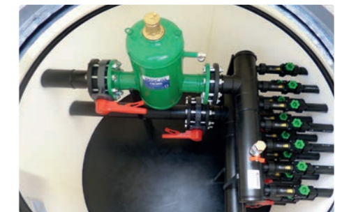
Chamber manifold with microbubble separator
