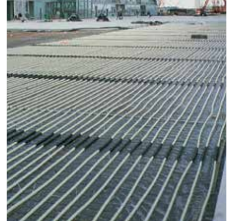
Roth industrial radiant heating
