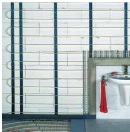
Roth wall heating
